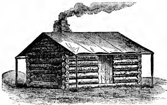
Winter hut for four men—the canvas roof protected by a fly which is fastened to a rail near the eaves.
